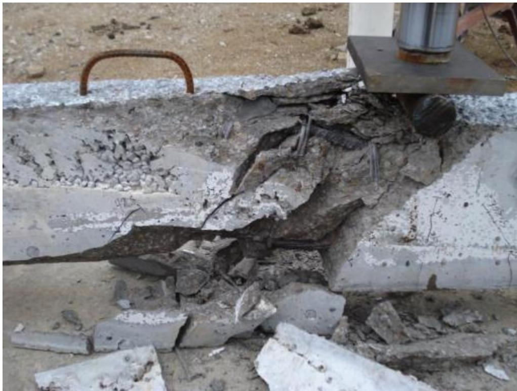
Figure 6.6: Failure of specimen NSC-2D
