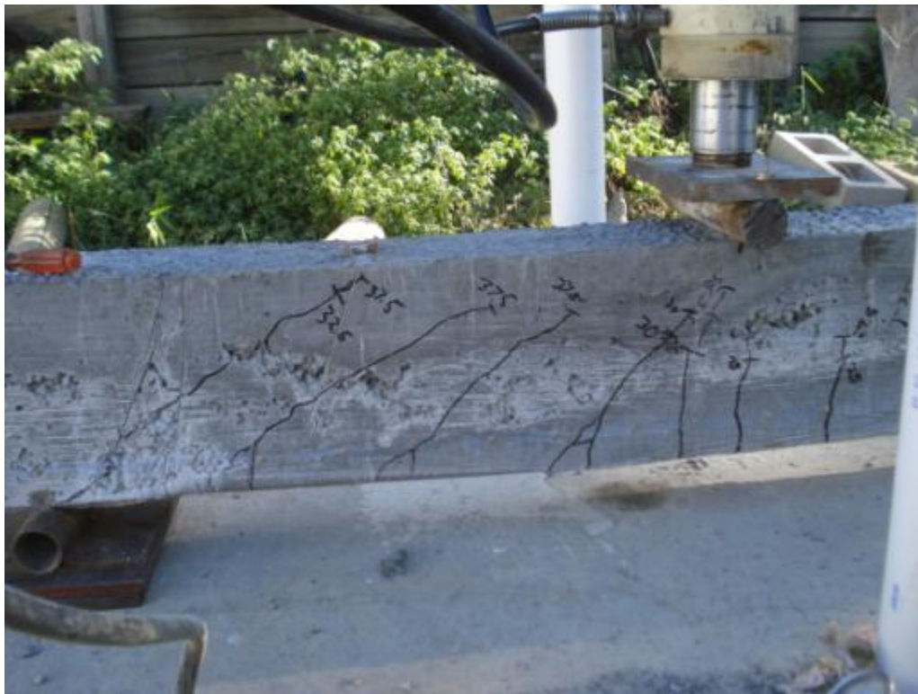
Figure 6.61: Cracking and failure of specimen HSC-3D
