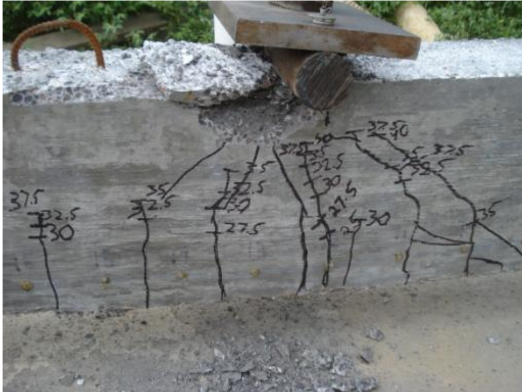
Figure 6.28: Failure of specimen NSS-3L
