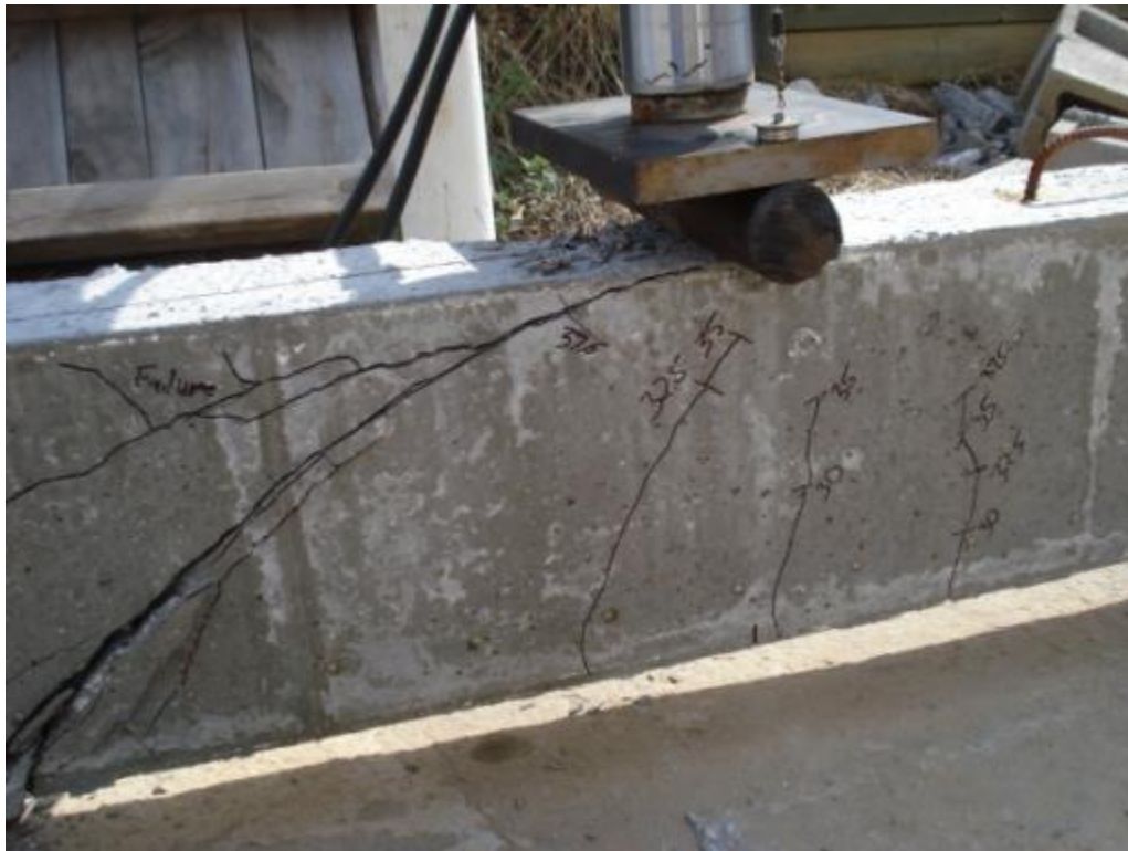
Figure 6.37: Shear cracking of specimen NSL-1D
