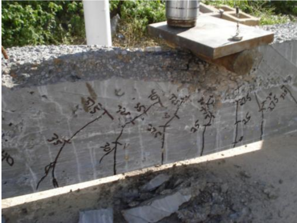
Figure 6.67: Cracking and failure of specimen HSC-4L
