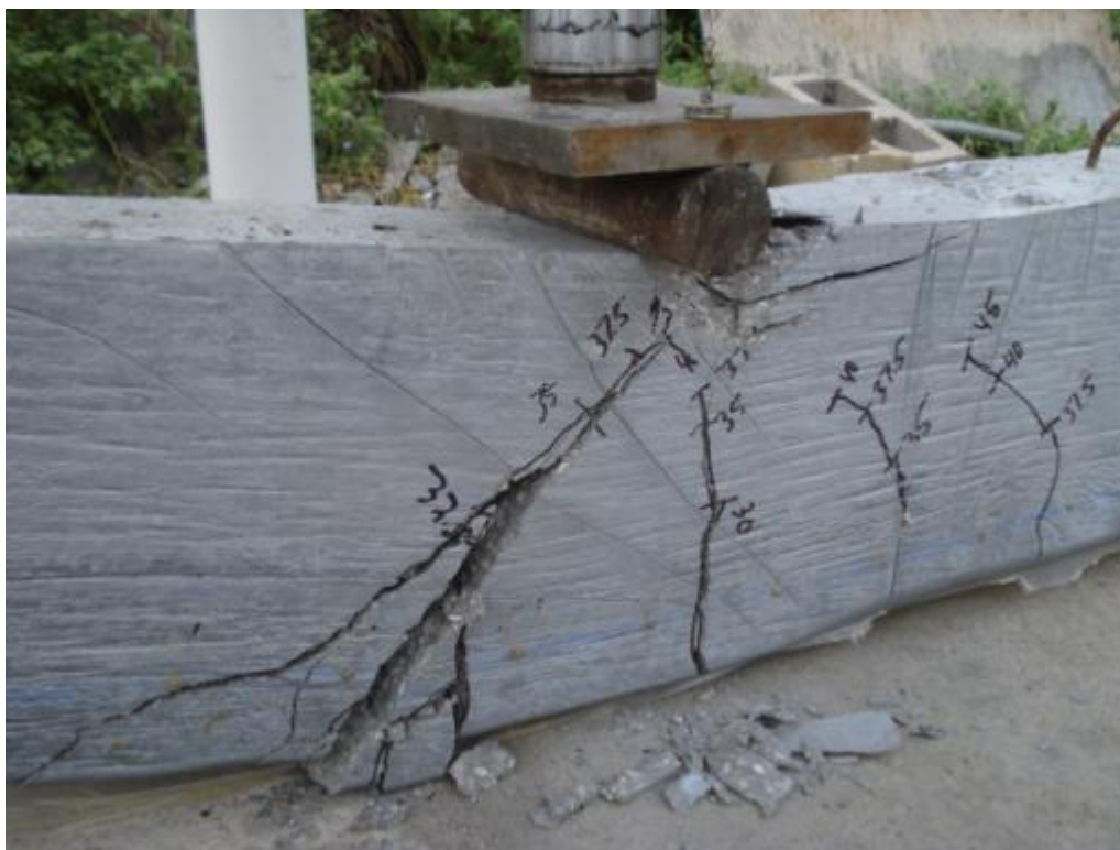
Figure 6.86: Cracking and failure of specimen HSL-1D
