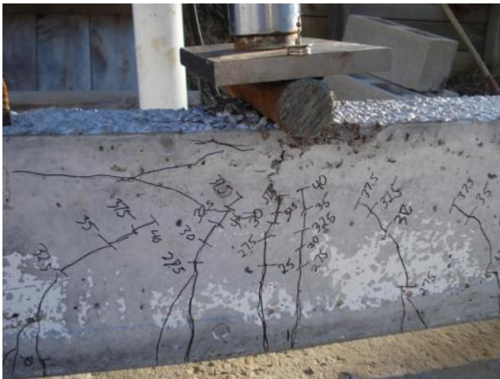
Figure 6.7: Cracking pattern of specimen NSC-2L
