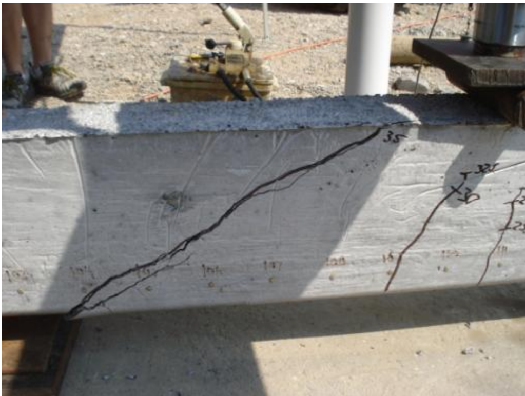
Figure 6.35: Shear cracking of specimen NSS-5L
