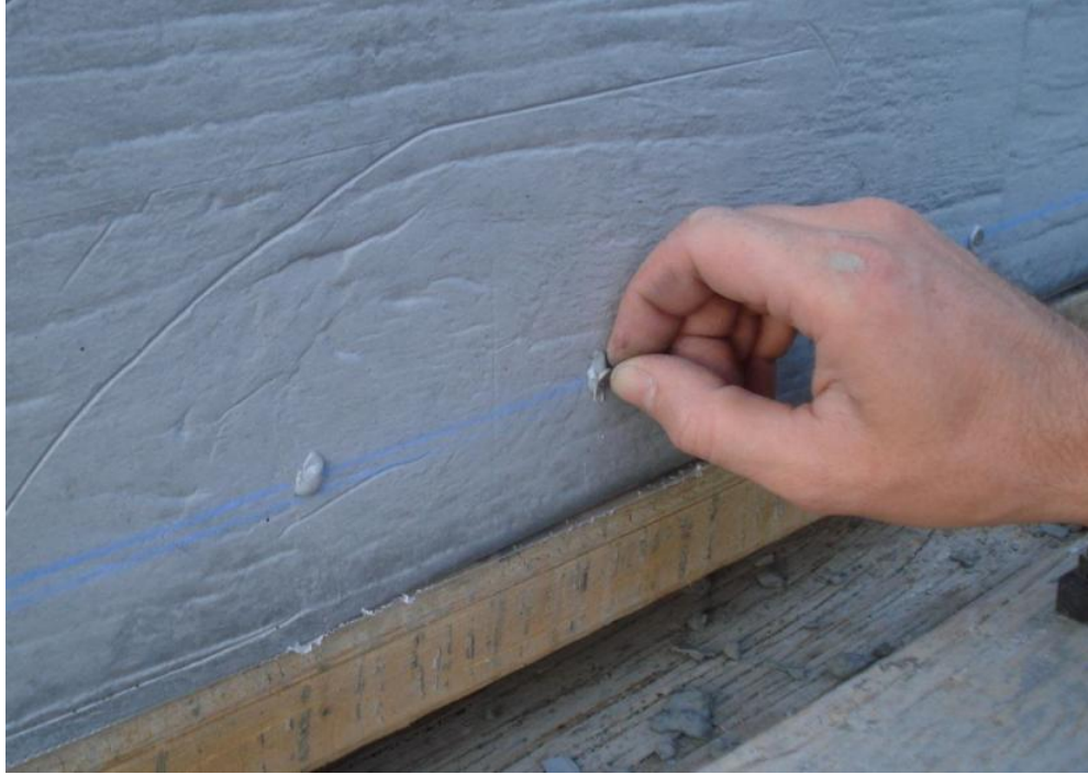
Figure 3.16: Placement of DEMEC points using epoxy
