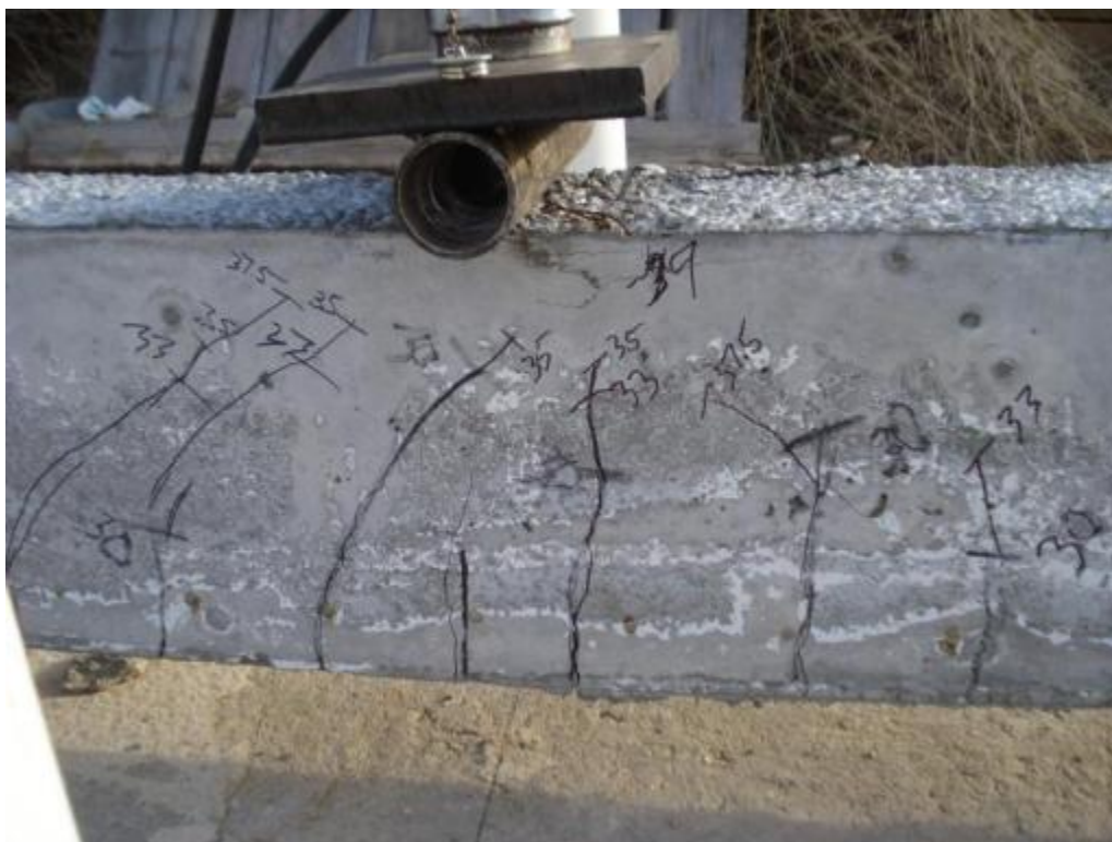
Figure 6.13: Cracking behavior of specimen NSC-4D
