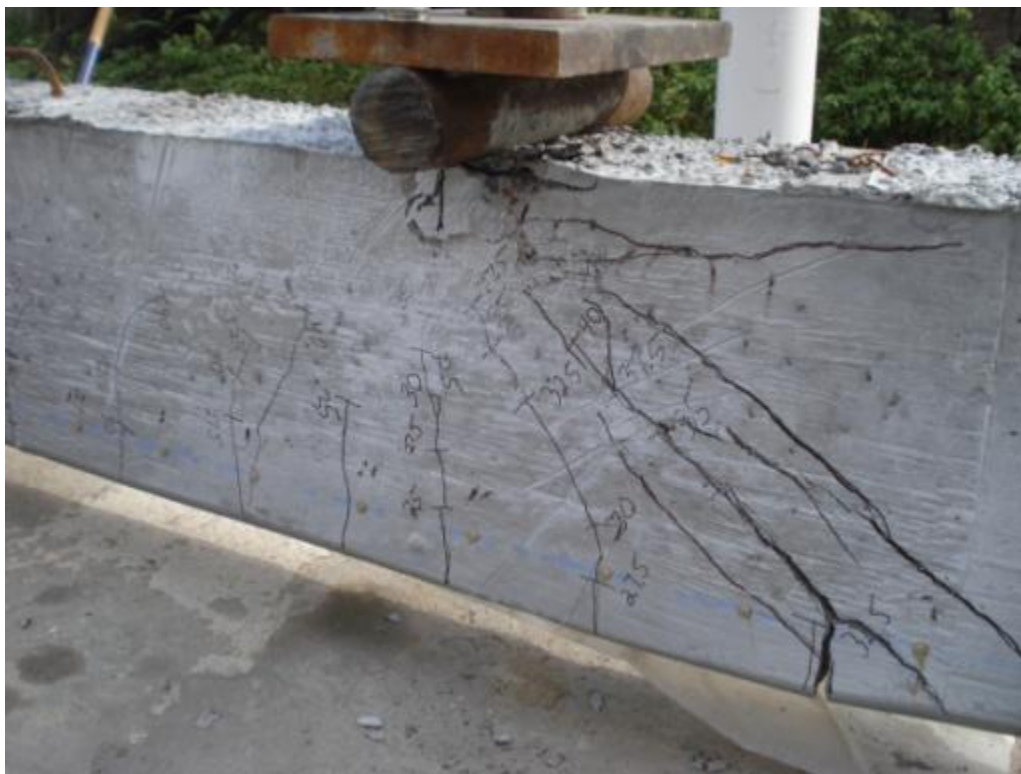
Figure 6.83: Cracking and failure of specimen HSS-4L
