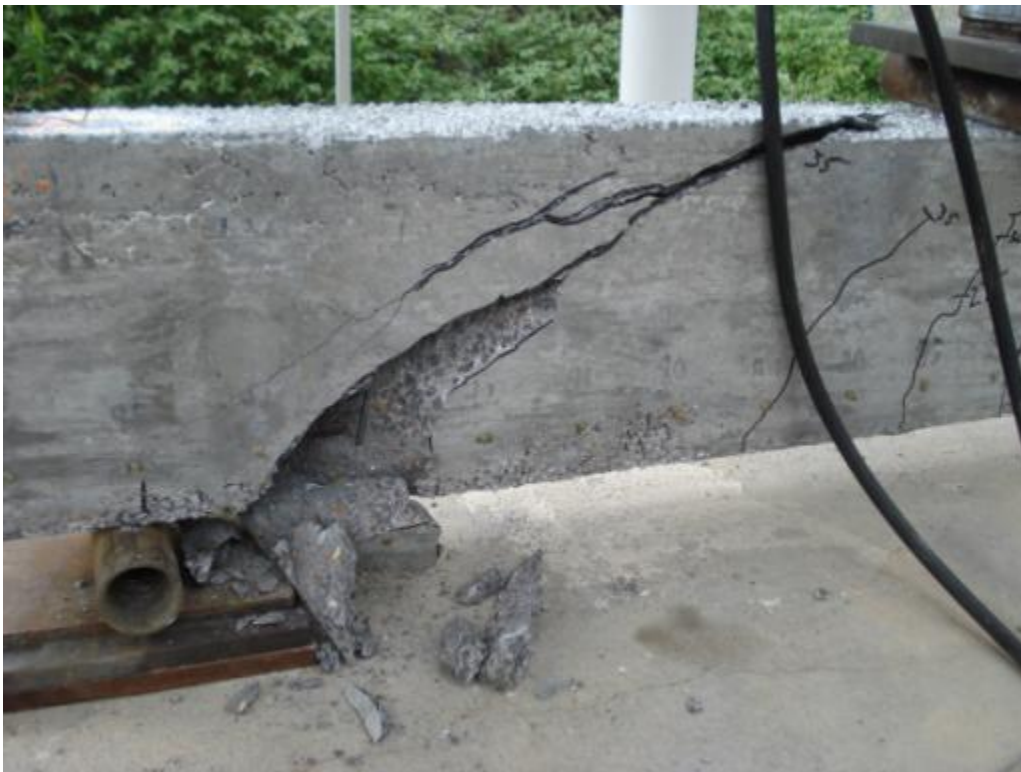
Figure 6.25: Shear failure of specimen NSS-3D
