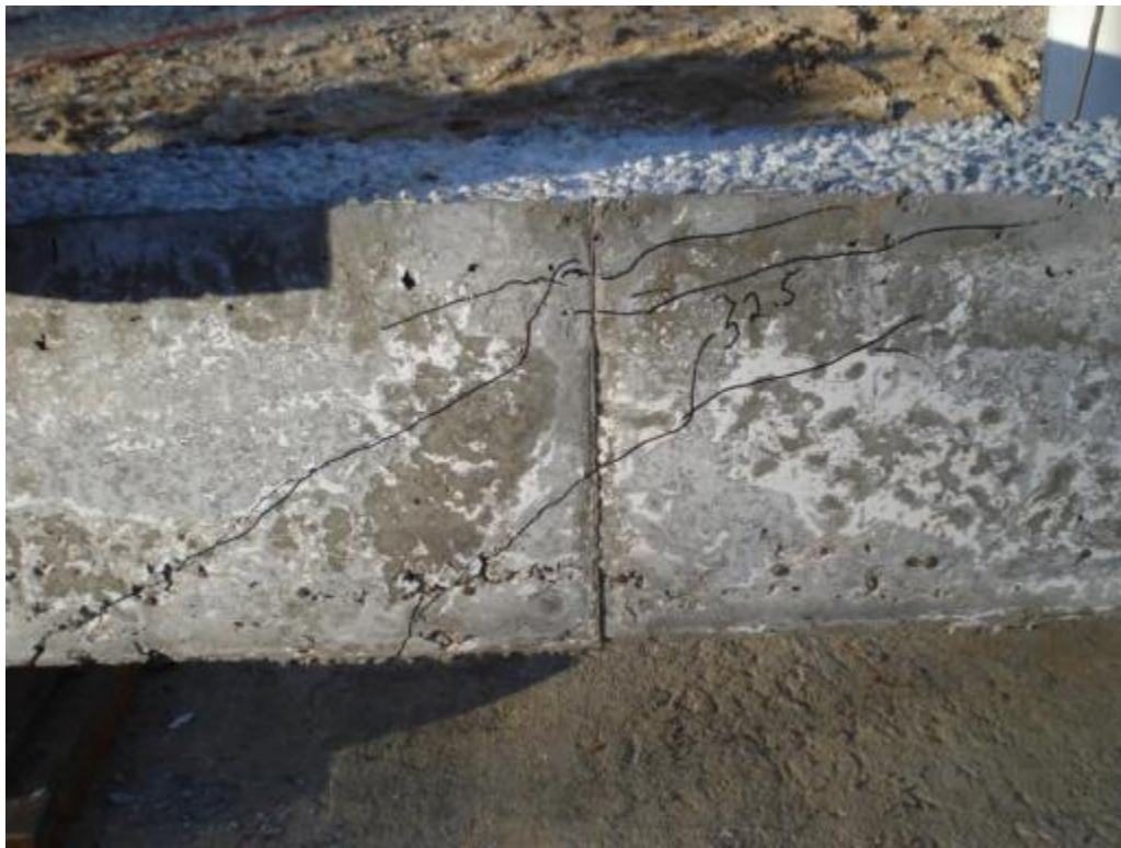
Figure 6.11: Shear cracking of specimen NSC-3L
