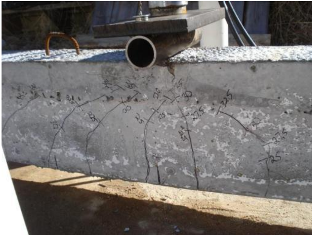
Figure 6.15: Cracking behavior of specimen NSC-4L
