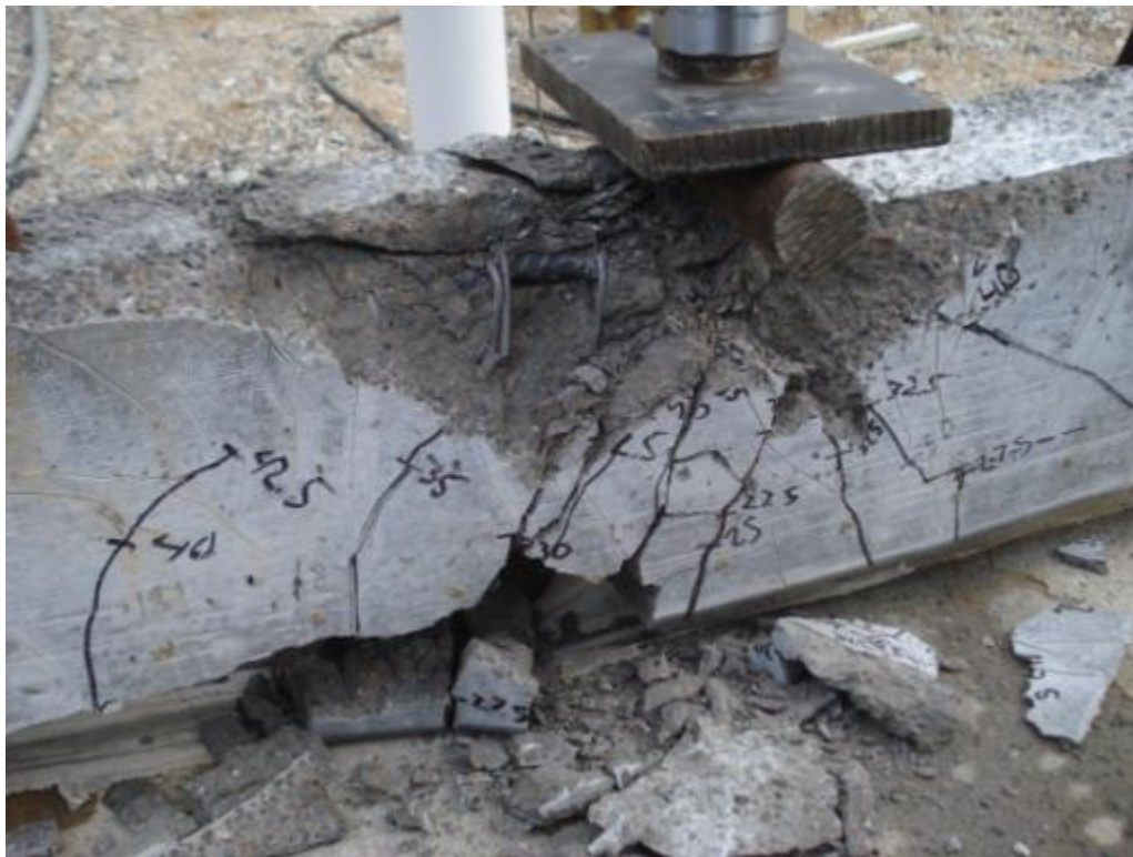
Figure 6.73: Cracking and failure of specimen HSS-2D
