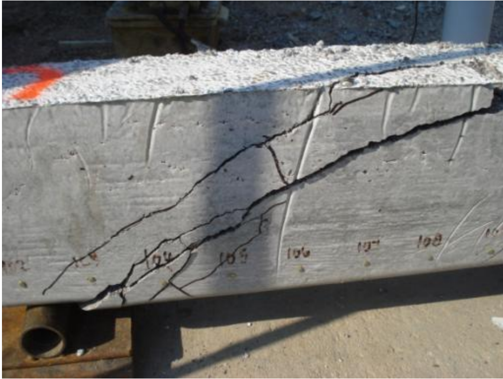
Figure 6.32: South side shear cracking of specimen NSS-4L
