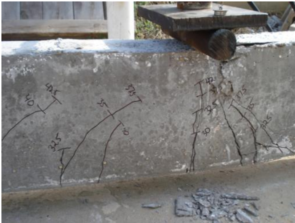
Figure 6.39: Cracking of specimen NSL-1L
