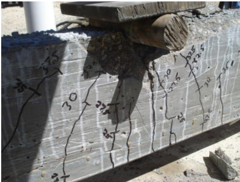
Figure 6.59: Cracking and failure of specimen HSC-2L
