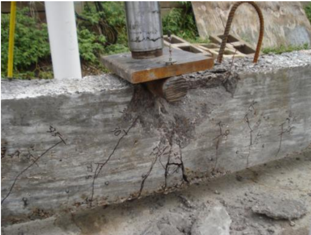
Figure 6.18: Cracking behavior and failure of specimen NSS-1D
