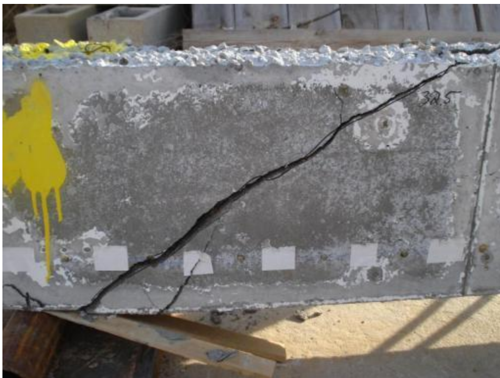
Figure 6.9: Shear cracking of specimen NSC-3D
