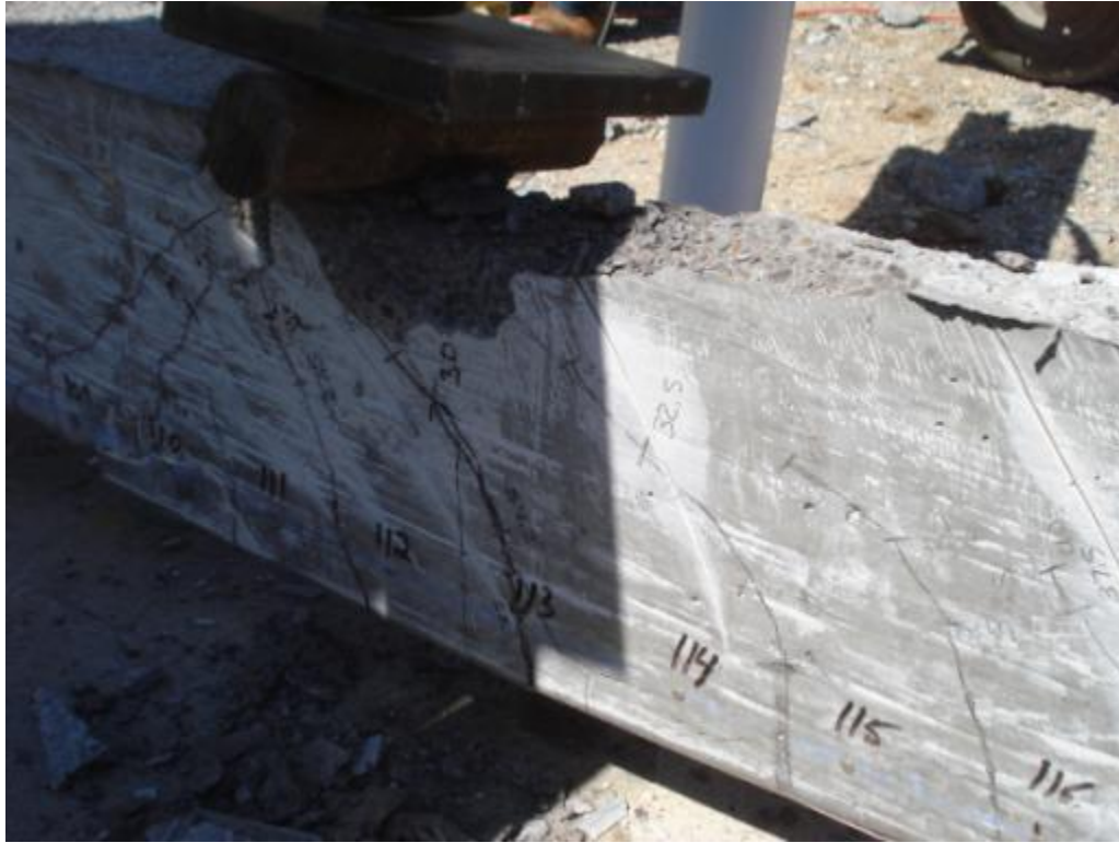
Figure 6.79: Cracking and failure of specimen HSS-3L
