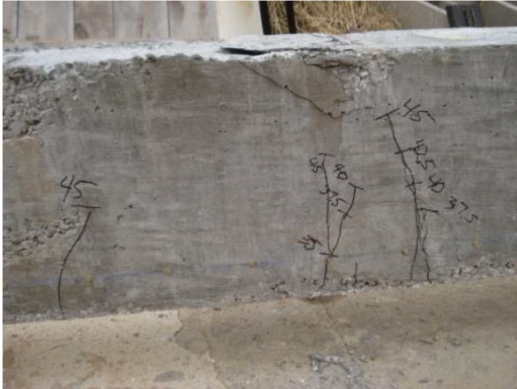
Figure 6.48: Cracking and failure of specimen NSL-3L
